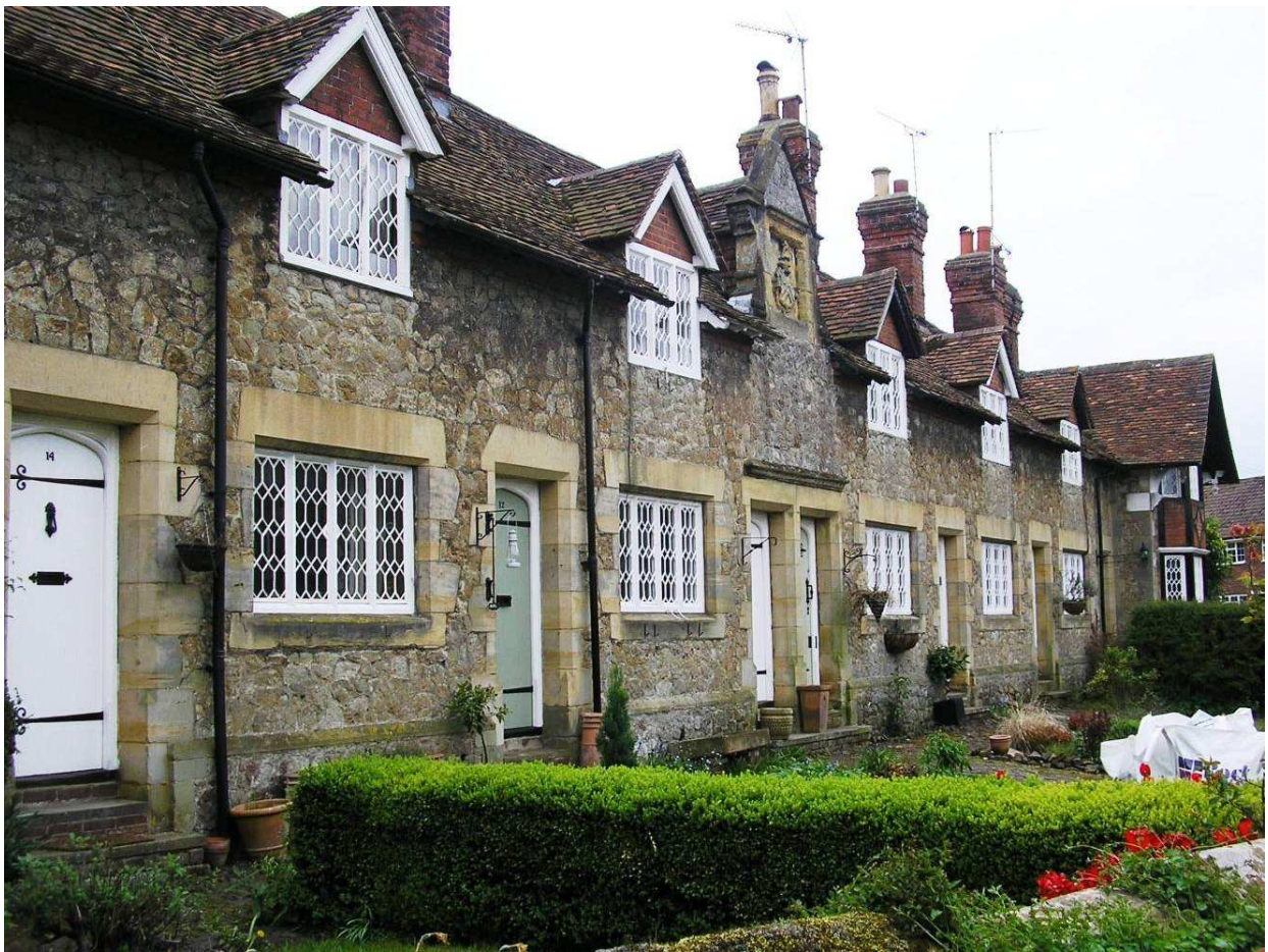
Former estate workers cottages, Chipstead Square
